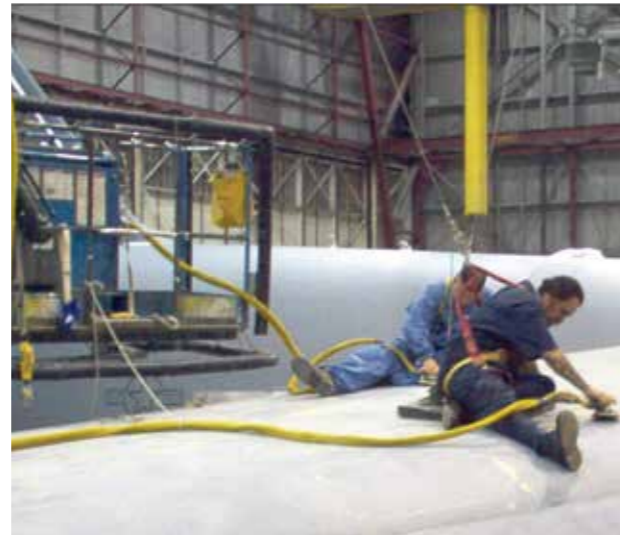
Workers sand a wing using hoses connected to a Clayton Distribution Module on an adjacent man lift.
